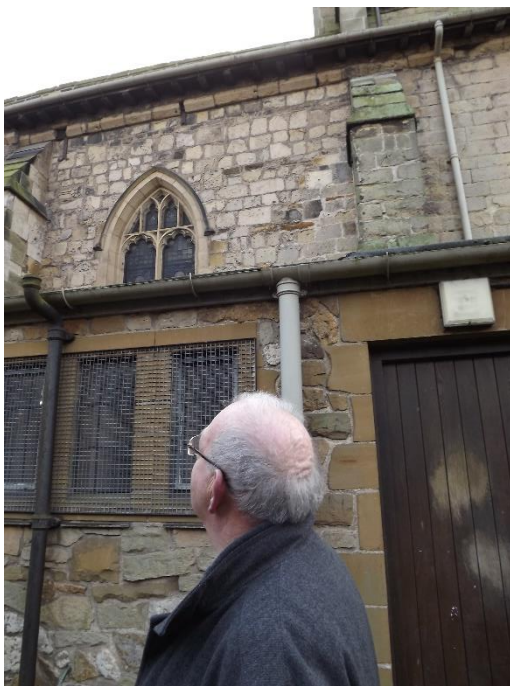
David Stanton viewing the 'new' cross. It's just to the left of the pointed window arch.
